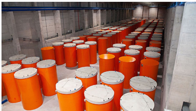
Spent Fuel Storage Facility (SFSF-2)
