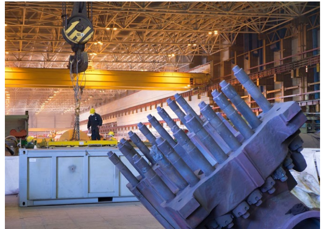
Radioactive waste pre-treatment site (Unit A1)
