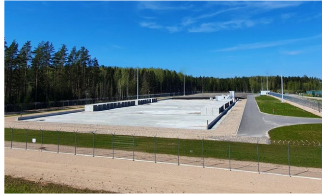
Very low level radioactive waste repository (under construction).
