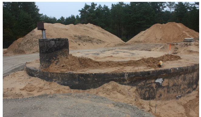
Decommissioning works of Maišiagala Radioactive Waste Storage Facility
