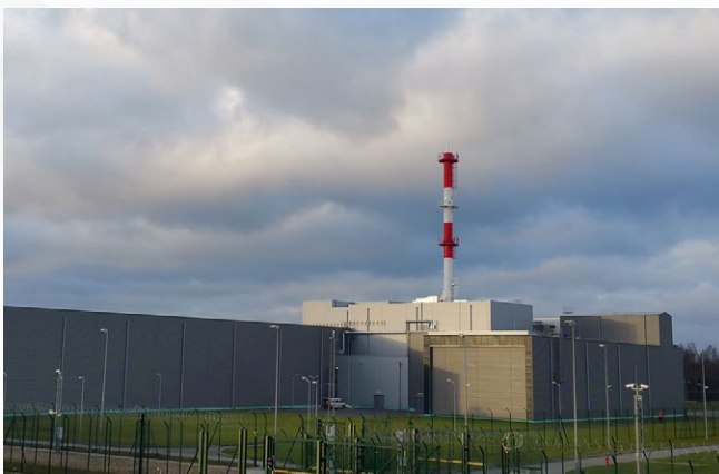
Facilities for treatment and storage of solid radioactive waste
